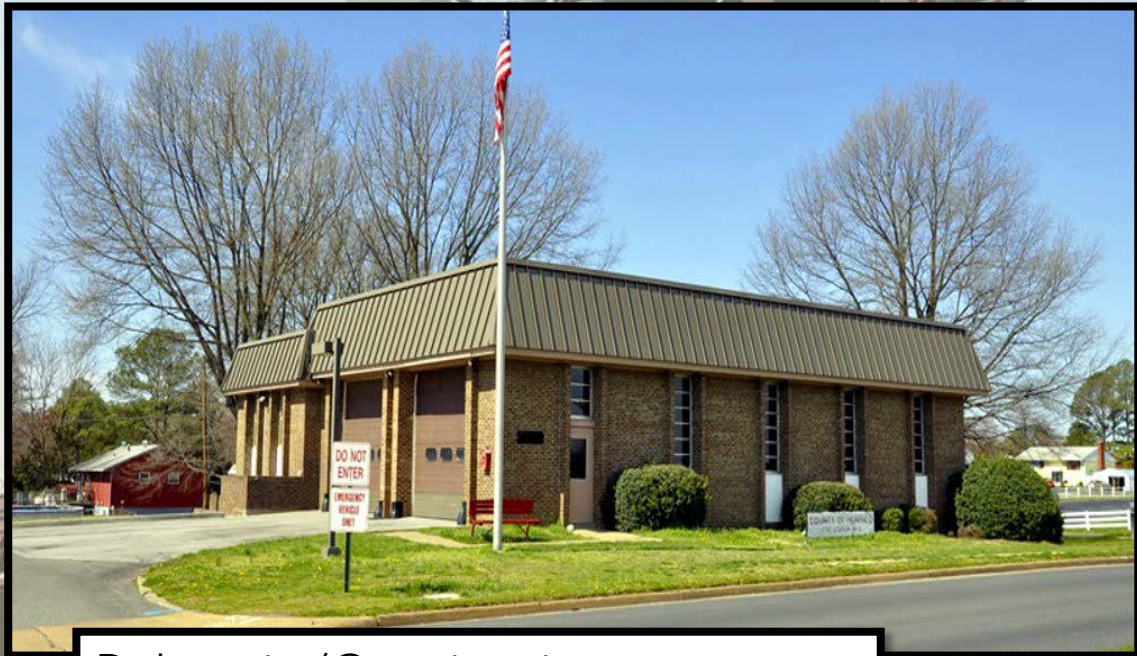
Relocate/Construct Firehouse #6 - Eastover Gardens
