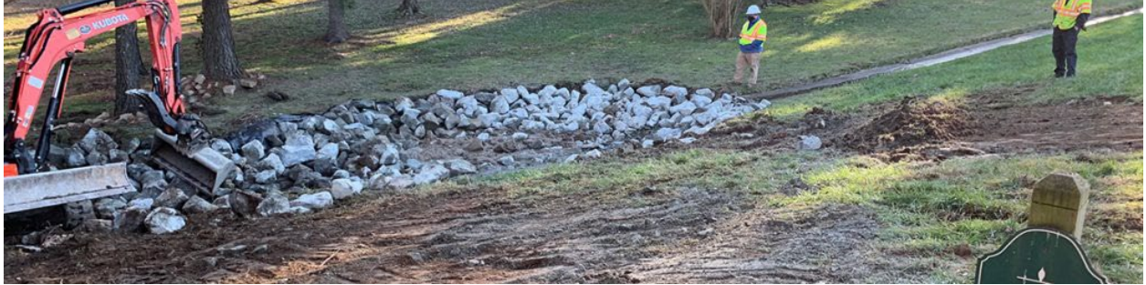
Drainage ditch work at Woodman Road
