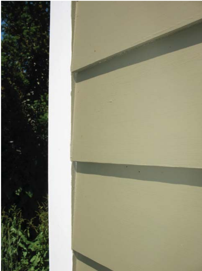
Fiber-cement siding was installed to meet a simple corner board.
