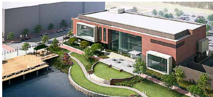
The Libbie Mill Library will open this fall on a 3-acre site in the Libbie Mill-Midtown development off Staples Mill Road. To check the progress of construction, go to henricolibrary.org/libbie-mill .
