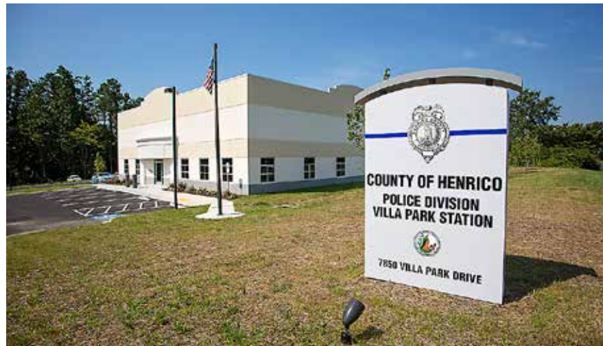
The Police Division opened the Villa Park Station at 7850 Villa Park Drive to enhance emergency response to central Henrico. The 10,000-square-foot precinct replaced a temporary station that had operated from Virginia Center Commons.
