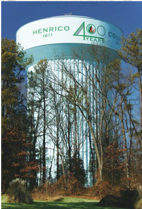
The Cox Road water tank, built in 1987, received its first new coat of paint last year. Crews used 1,500 gallons of paint to refinish the tank, which stands 160 feet above the county's western skyline and holds 2 million gallons of water.
