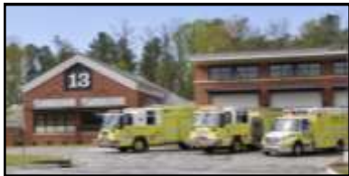
Firehouse 13, 12491 Church Road
