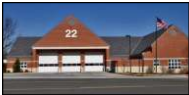
Firehouse 22, 3790 Westerre Parkway
