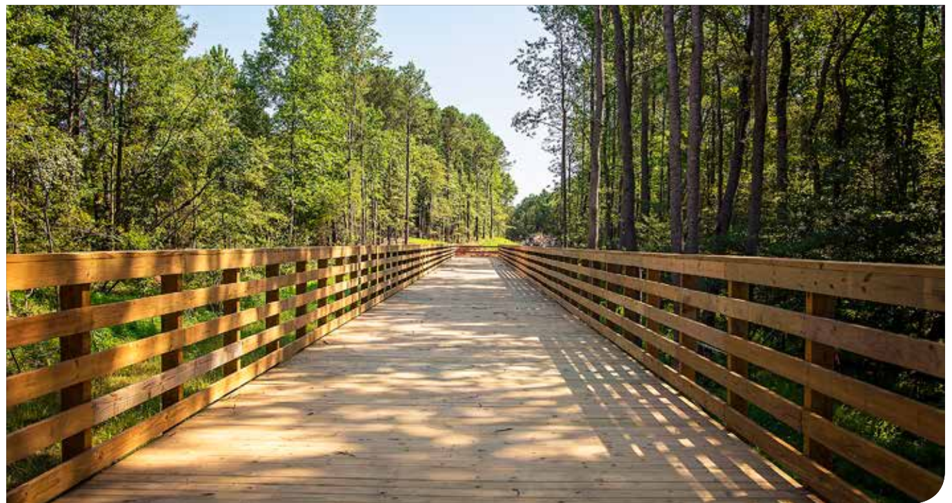
Bicyclists should be able to pedal the full 52 miles of the Virginia Capital Trail — including this bridge near Henrico's Four Mile Creek Park — by late September.
