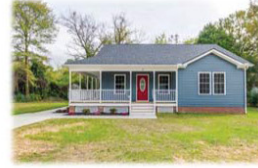
Affordable home constructed
