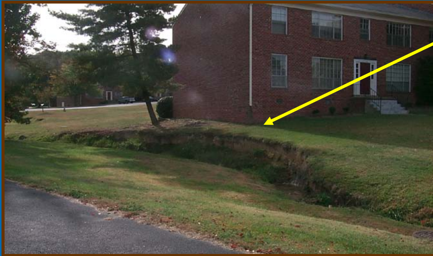
Erosion endangering building foundations
