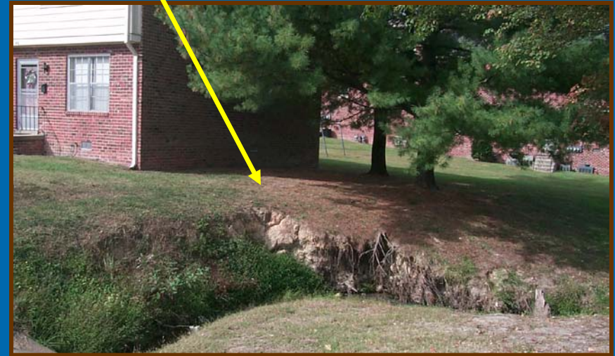
Erosion endangering building foundations
