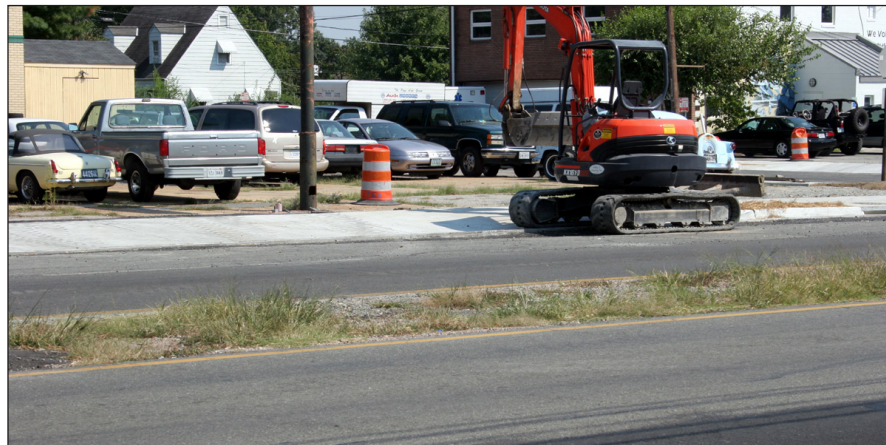
Figure 13: Property owners expressed disappointment with ongoing road construction
