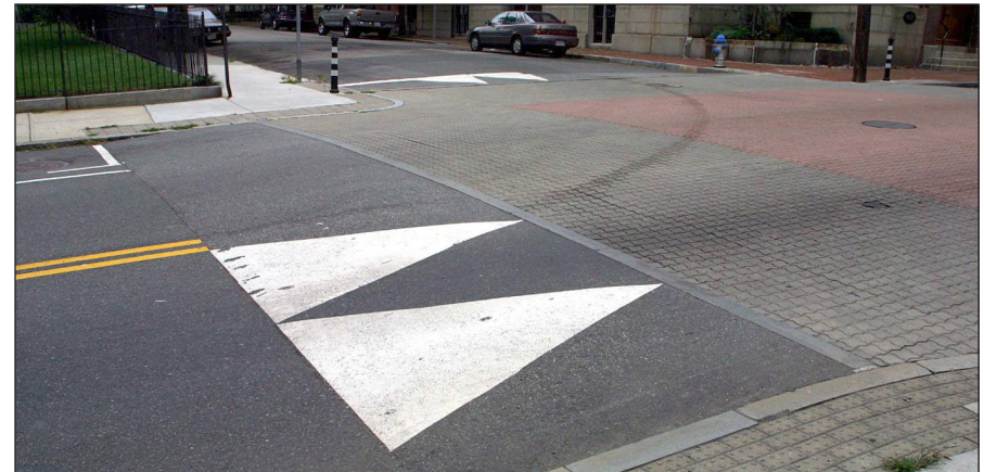
Figure 25: Raised intersections will improve mobility and access for all modes of traffic
