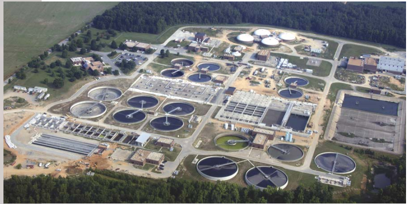
Henrico's steady growth requires quality infrastructure to sustain it. In FY 06, the newly expanded Water Reclamation Facility received approval to treat up to 75 million gallons per day; currently, the facility handles an average of 43 million gallons per day.
