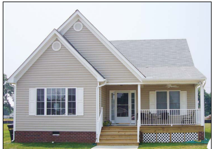
MH/MR Residential Services built a new group home for several clients in FY 07. The Shurm Heights facility includes four bedrooms, two-and-a-half baths and ADA-compliant living quarters for its adult residents.
