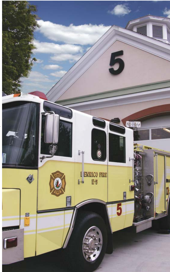
The new Fire Station 5 in Lakeside nearly doubles the size of its predecessor and features a more accessible apparatus bay.
