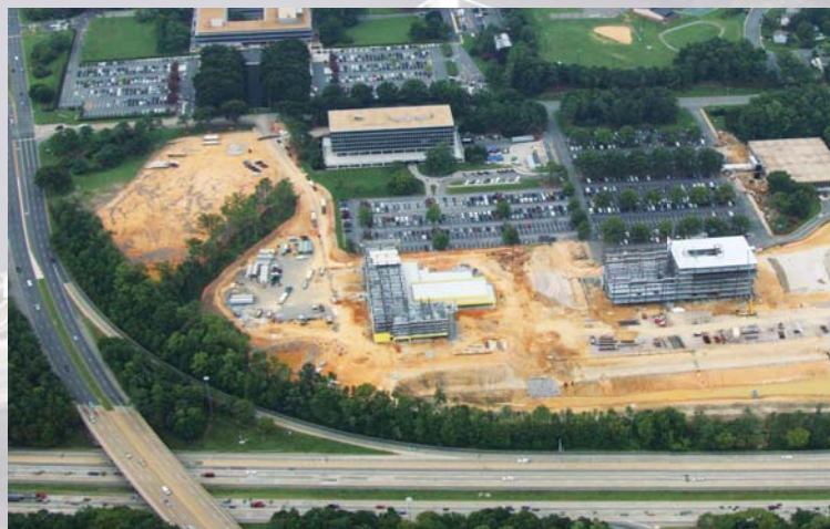
When completed, the Reynolds Crossing site will feature 71 acres of upscale office and retail development, including a Westin Hotel, Bookbinder's restaurant and facilities for Philip Morris USA and Bon Secours Health System.
