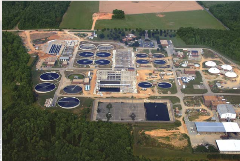
Henrico's water treatment plant was recognized for its operations excellence by the Virginia Department of Health last year.
