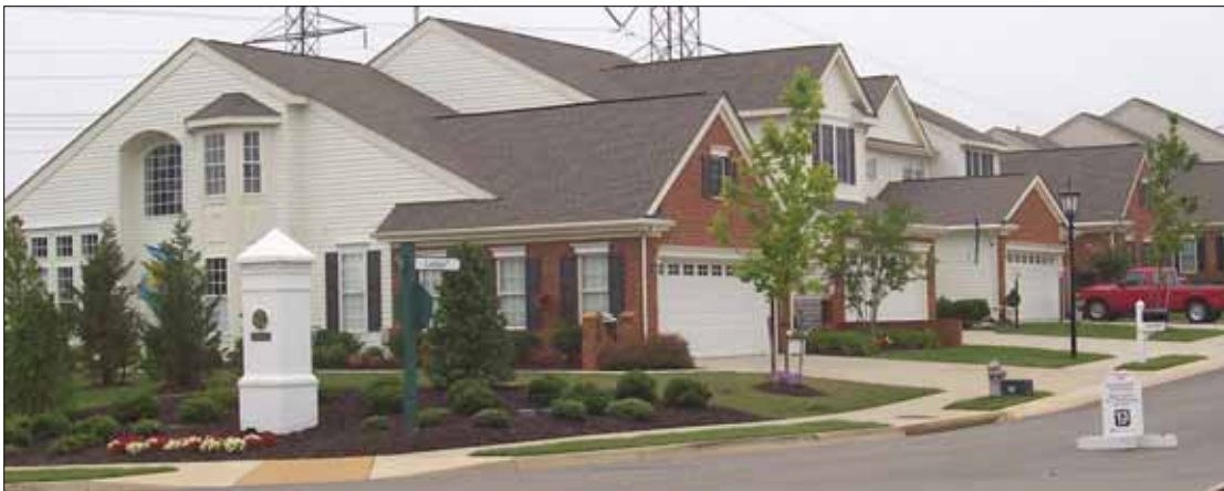
The entrance into this Henrico County, VA neighborhood is celebrated with landscaping, signage, sidewalks, etc.
