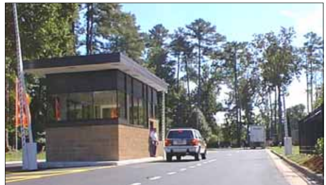
A security gate at this site in Virginia Beach, VA controls access into the facility.
