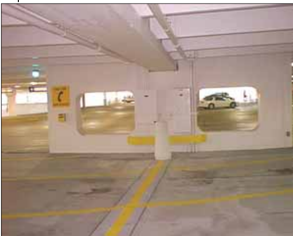
The parking garage at MacArthur Mall in Norfolk, VA has cut out areas in the concrete wall separators. This allows light to pass through, provides visibility to various sections of the garage and allows sound to travel. Emergency phones are also available and the garage is very well lit.
