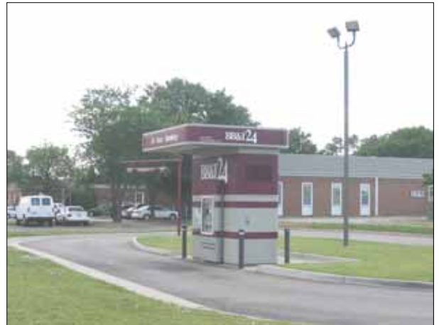
Users of this ATM in Virginia Beach, VA have opportunities to view around them. No hiding places have been created with landscaping or other buildings. The surrounding area can also see this area and what is going on.
