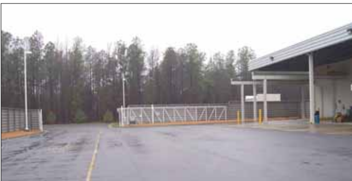
Fencing has been provided around the loading area in this warehouse in Henrico County, VA. Lighting is also in place.
