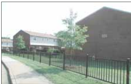
This fence shows public and semi-private areas, controls access, and offers visibility from a Henrico County, VA street.
