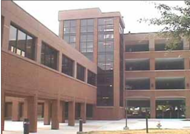
This parking deck in Henrico County, VA is very open and visible. Using less concrete adds to the open feeling within the deck. Surveillance is possible to the stairwell and elevators with glass walls in place.
