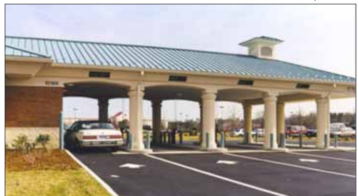
The ATM at this credit union in Henrico County, VA has been located in the first drive-through aisle. This design provides safety for the customer and employee. The customer can remain in the safety of his or her vehicle, and the employee can make deposits and withdrawals from a secure area inside the bank.
