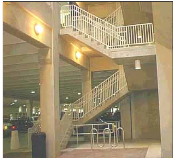
The parking garage in MacArthur Mall in Norfolk, VA was designed with CPTED strategies in mind. This stairwell is open, well lit and very visible. It is used as a design feature by its location and layout.
