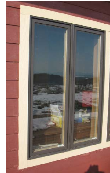
These aluminum-clad wood casement windows may be appropriate when a less traditional appearance is sought.
