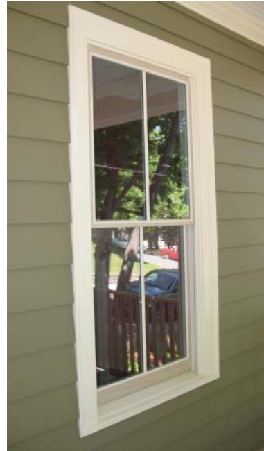
New windows should be accompanied by appropriate trim as seen in this traditional vinyl-clad wood, double-hung window example.
