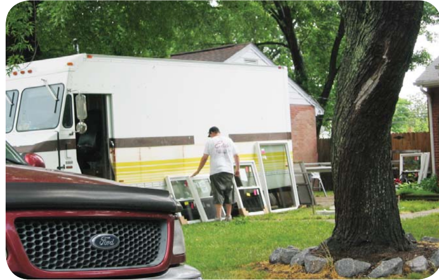
At this house, in the east end of Henrico County, contractors were able to park their work truck in the driveway and were given ample outdoor workspace.
