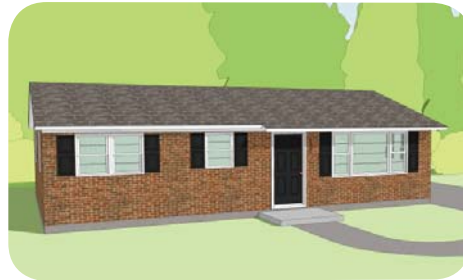
EXISTING FRONT VIEW
