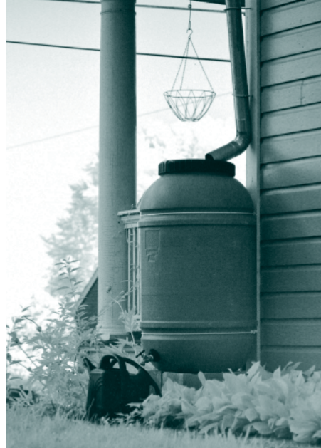
A rain barrel collects water from a downspout for use in the garden.
