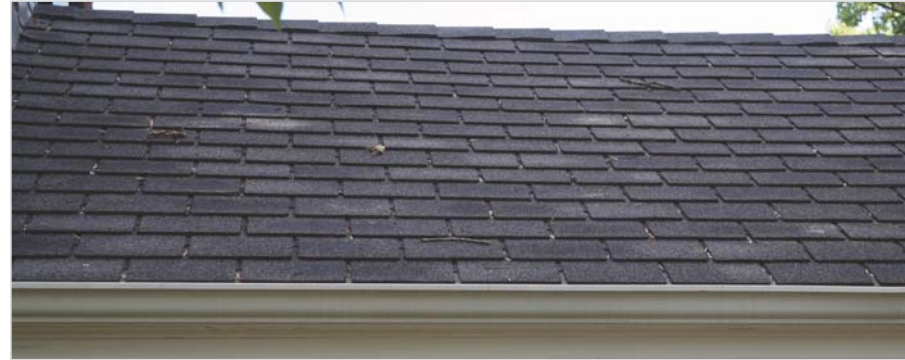
This laminated shingle roof provides three-dimensional visual interest.
