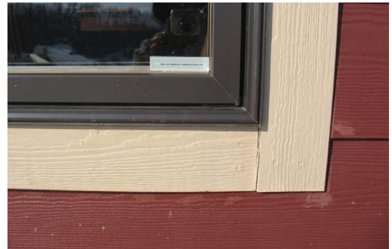
Wood-grained fiber-cement trim complements the similarly textured siding.
