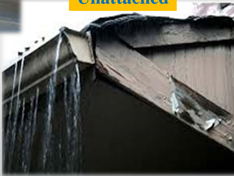
Gutter Unattached
