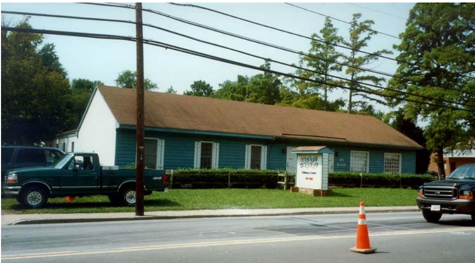
A car is parked in the grass because of lack of parking spaces at the day care facility. Creating on-street parking here will help this parking problem.
