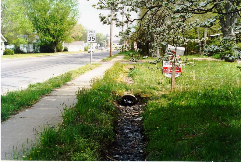
A drainage swale along East Williamsburg Road
