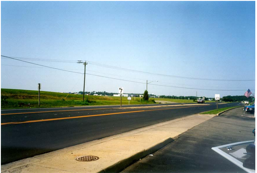
View west of west gateway, and position of relocated merge lane
