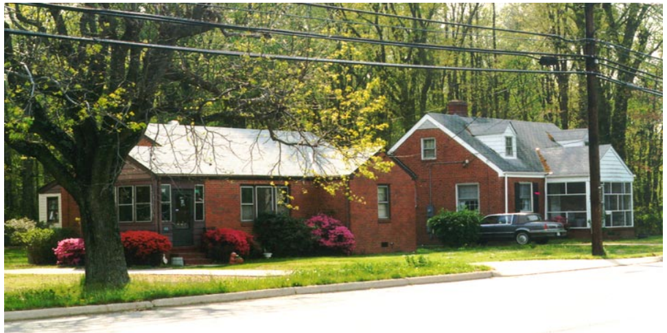
Residential area along East Williamsburg Road
