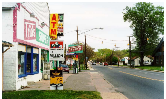
Example of a building with a new gable roof - with the gable oriented toward the street rather than the building's sides
