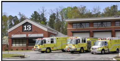
Firehouse 13 , 12491 Church Road
