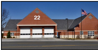
Firehouse 22 , 3790 Westerre Parkway
