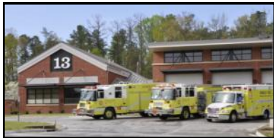
Firehouse 13 , 12491 Church Road
