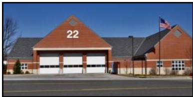
Firehouse 22 , 3790 Westerre Parkway
