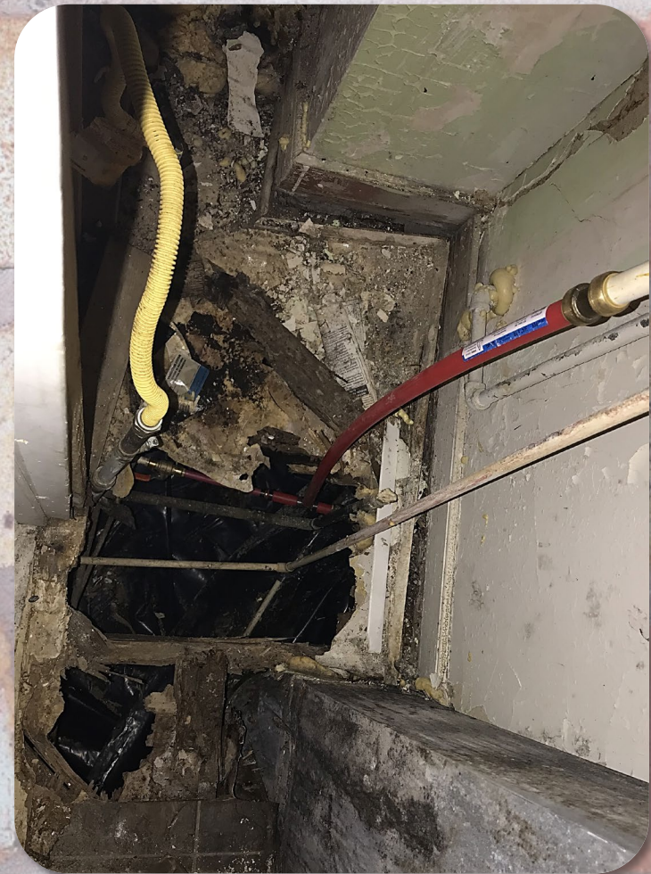
Rotten/Missing floors
