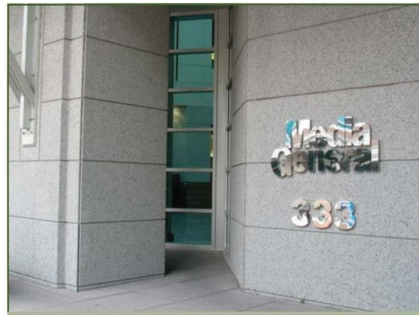
An example of building identification signage on a high-rise building.
