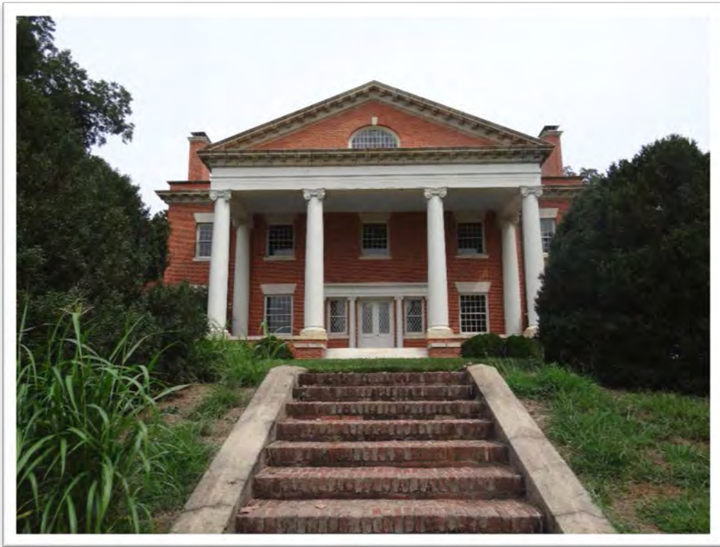
East façade of Manor House facing the river
