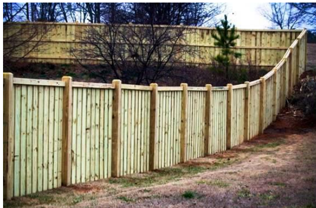
Figure 5406A: Fence with Finished Side Facing Out
