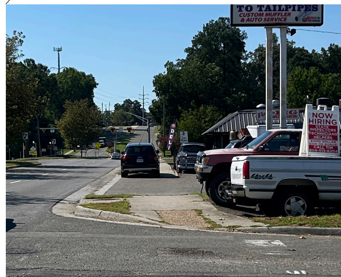
Large curb cuts interrupt sidewalks
