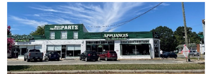
Adkins Furniture Store, 1941 (top) and Lakeside Appliance (bottom).
