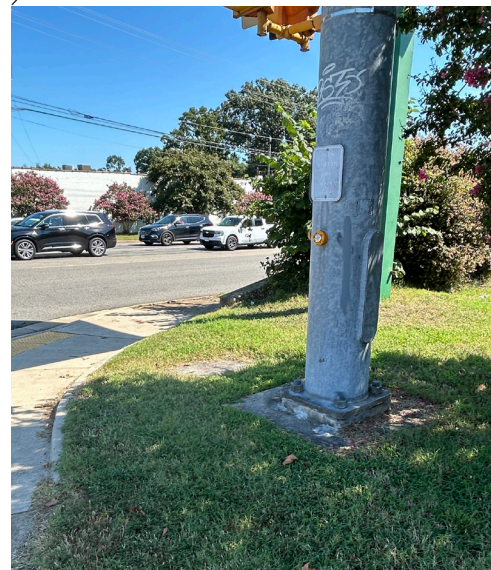
Inaccessible button and handicap ramp with no striped crosswalk on Dumbarton
