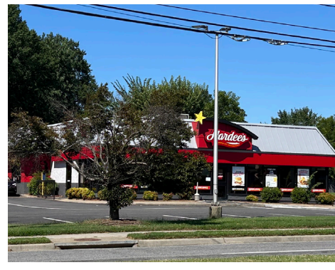
Non-Contributing Even though this frontage has a sidewalk, the fact that there is a parking lot between the building and the street and the building has dark tinted windows means it is non-contributing.
