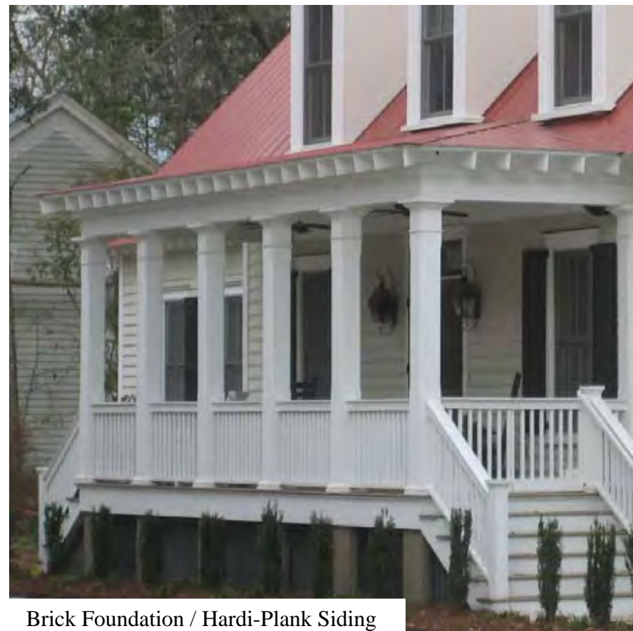
Brick Foundation / Hardi-Plank Siding
