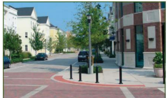
Roll-down curbs provide for increased maneuverability of larger vehicles.
