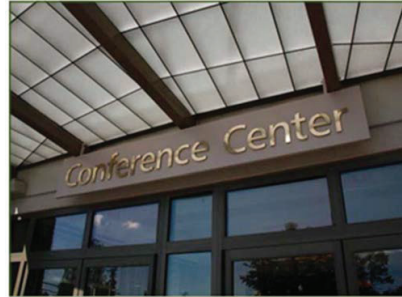
Low rise buildings may have one building identification sign per public entrance lobby. Maximum size is 4 square feet.
