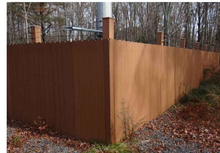
ILLUSTRATION: FENCING TO BE CONSTRUCTED OF SOLID RECYCLED PLASTIC, ENGINEERED PLASTIC, COMPOSITE OR OTHER SIMILAR MATERIALS AS MAY BE APPROVED BY THE PLANNING DEPARTMENT.
