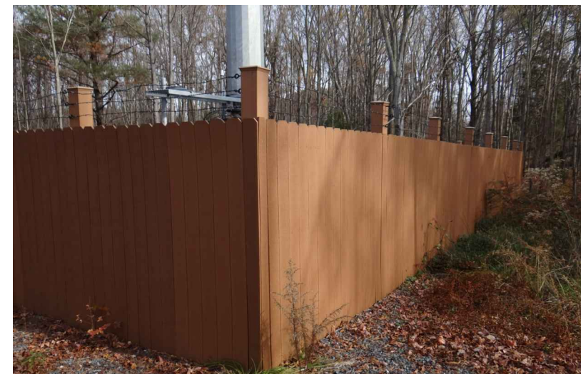
ILLUSTRATION: FENCING TO BE CONSTRUCTED OF SOLID RECYCLED PLASTIC, ENGINEERED PLASTIC, COMPOSITE OR OTHER SIMILAR MATERIALS AS MAY BE APPROVED BY THE PLANNING DEPARTMENT.
